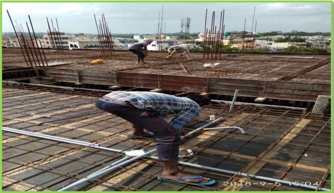
4 TH FLOOR SLAB BAR BENDING WORK CUM ELECTRICAL WORK
