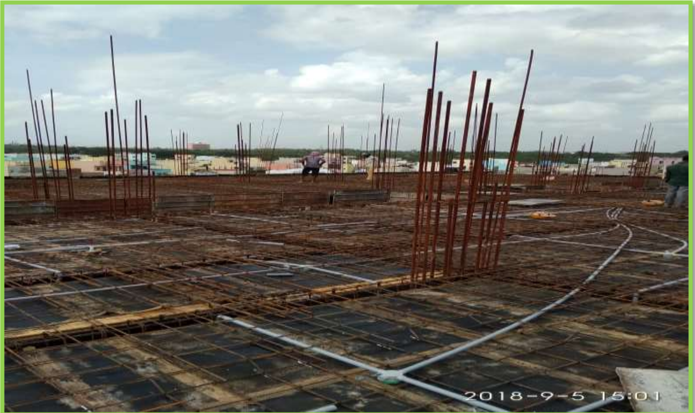
4 TH FLOOR SLAB BAR BENDING WORK CUM ELECTRICAL WORK
