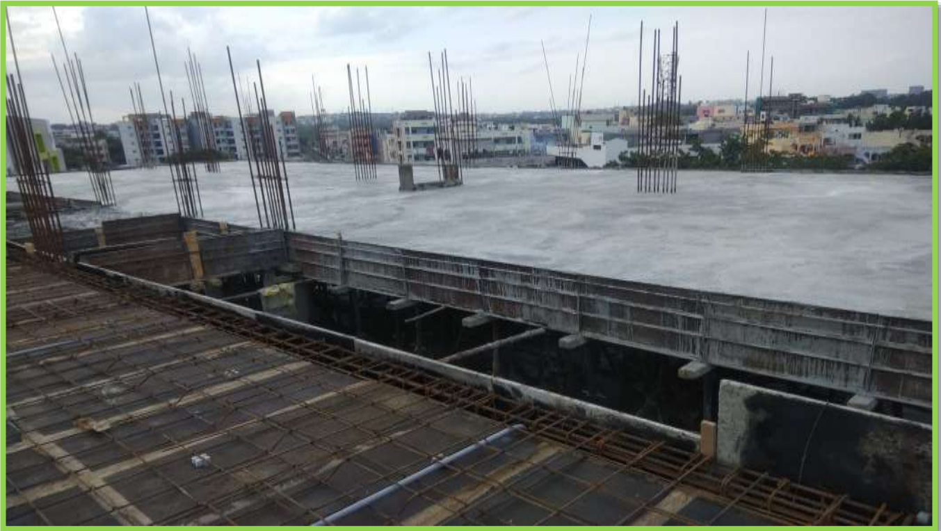
4 TH FLOOR SLAB CONCRETE WORK
