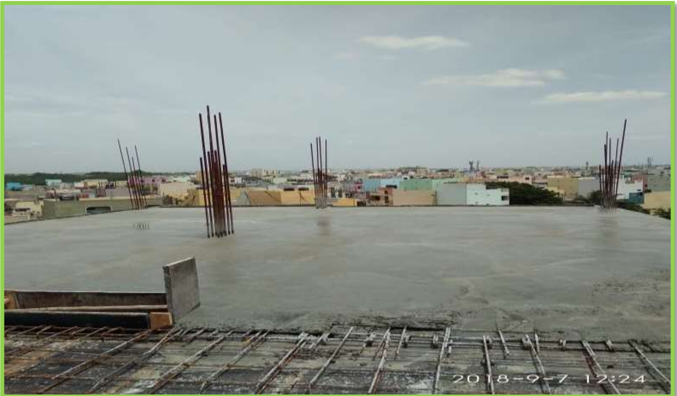
4 TH FLOOR SLAB CONCRETE WORK
