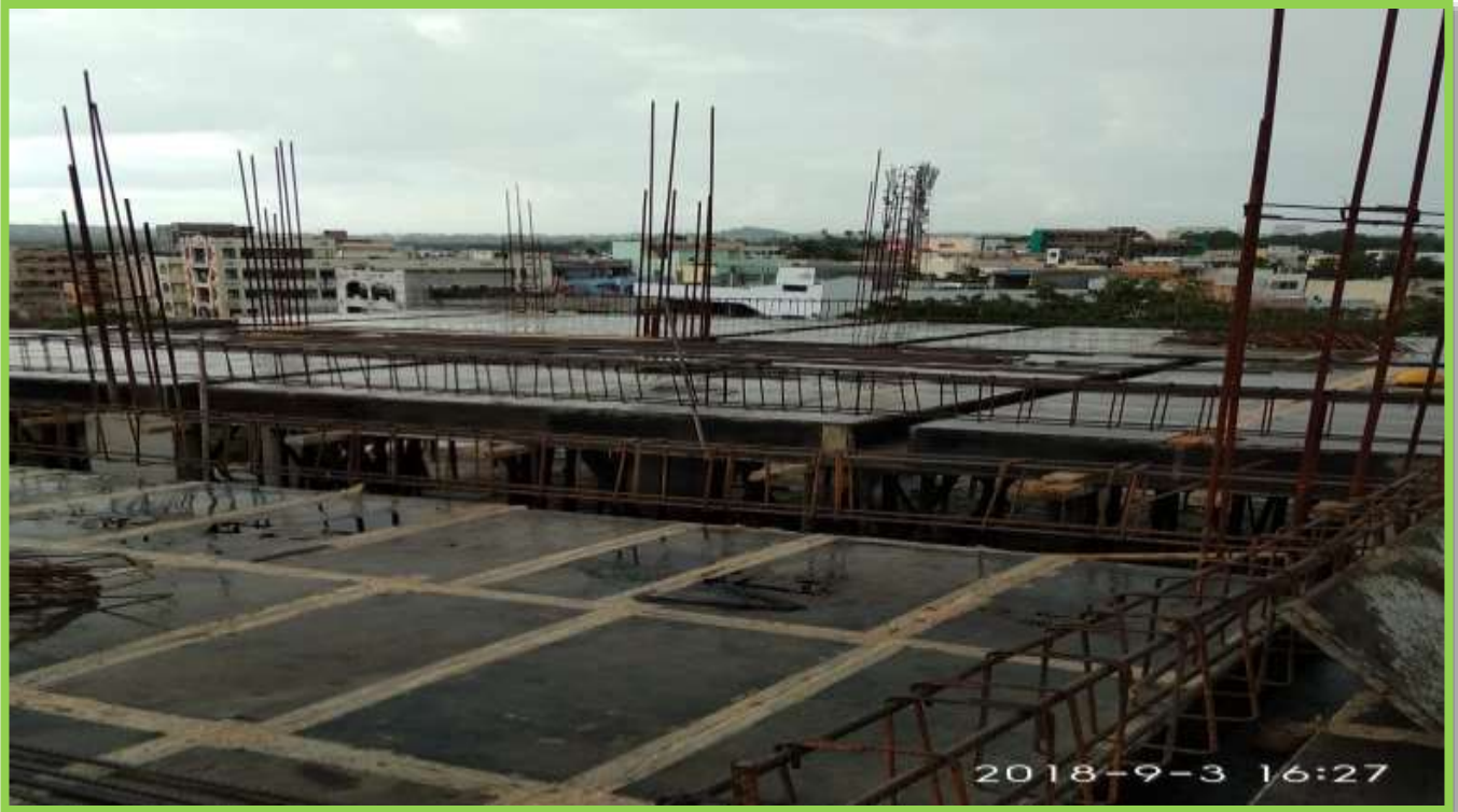
4 TH FLOOR SLAB SHUTTERING WORK
