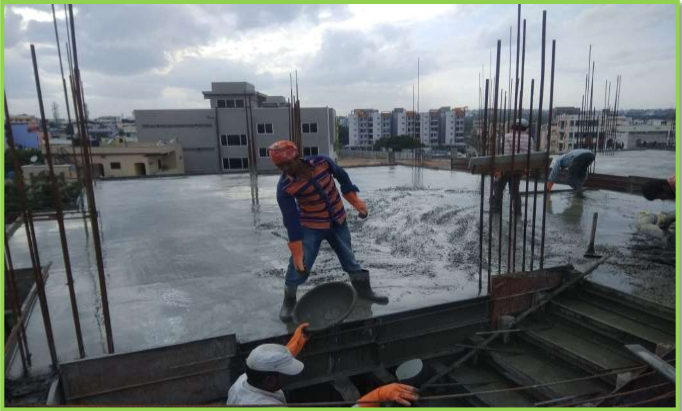
4 TH FLOOR SLAB CONCRETE WORK
