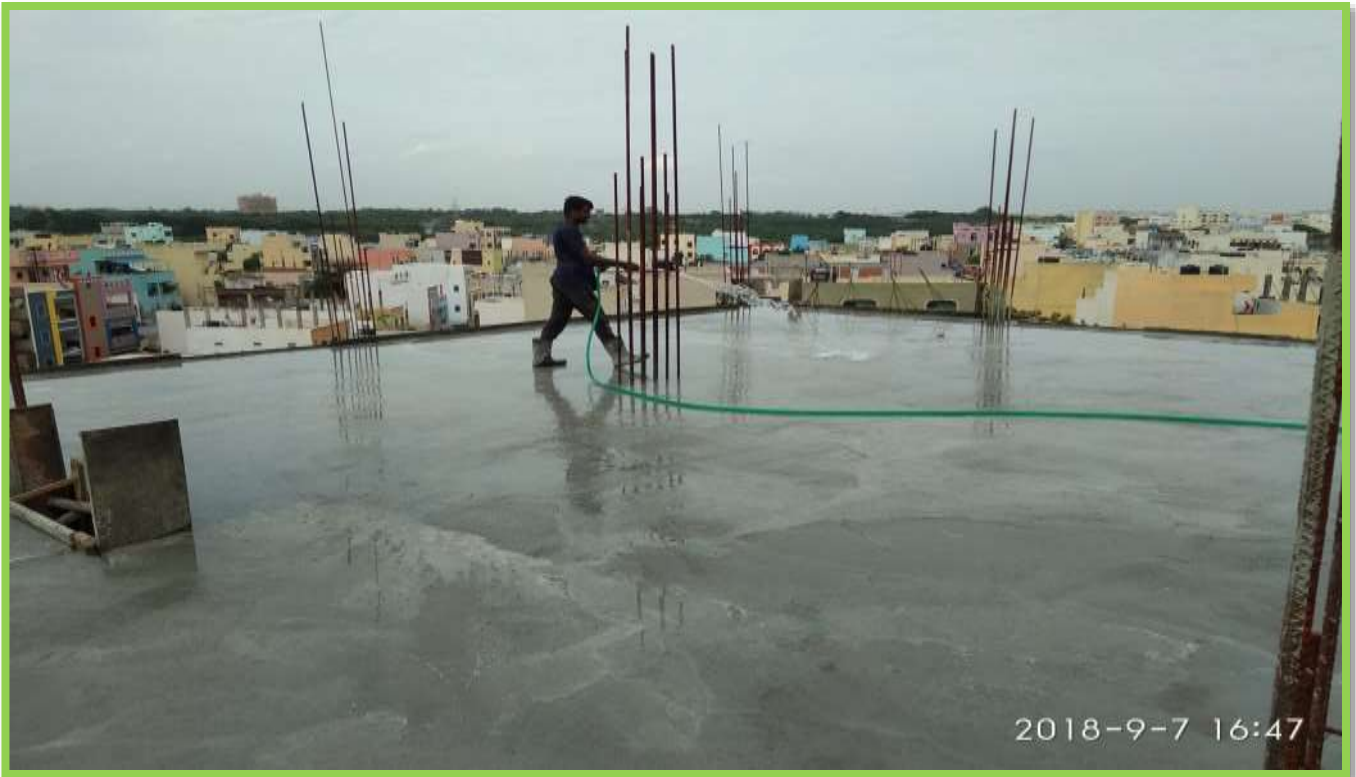
4 TH FLOOR SLAB CONCRETE WORK
