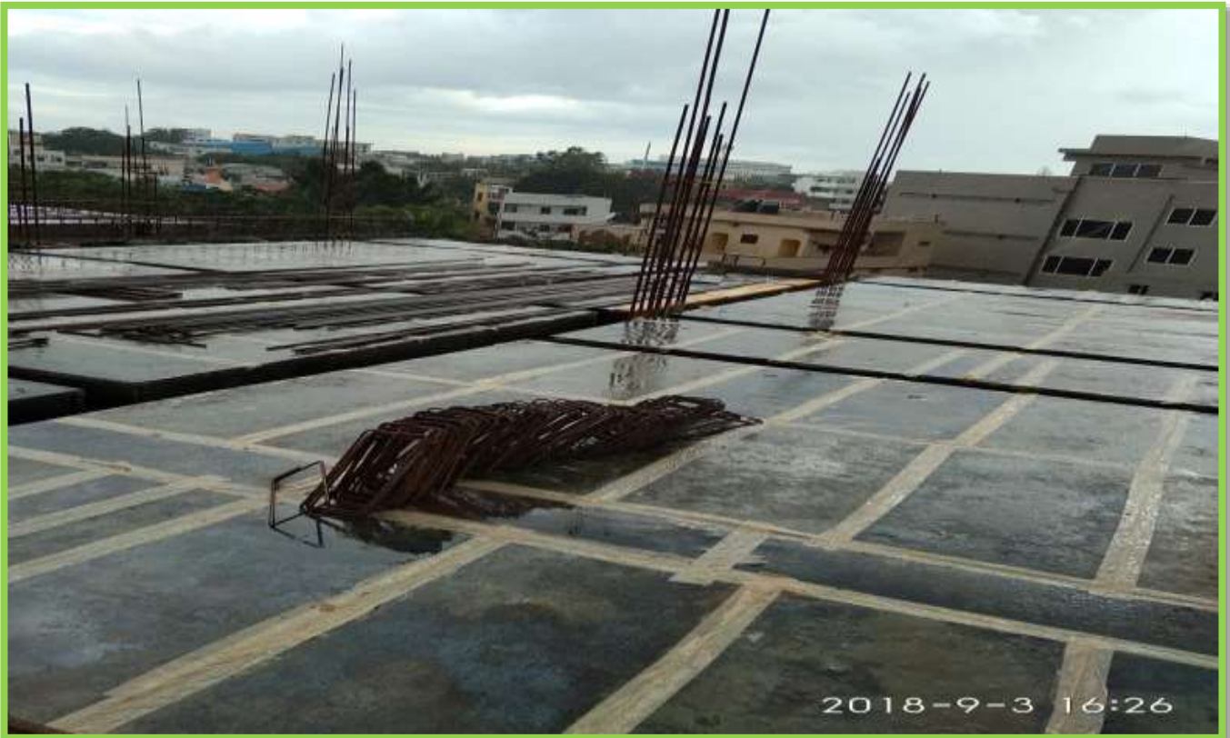
4 TH FLOOR SLAB SHUTTERING WORK
