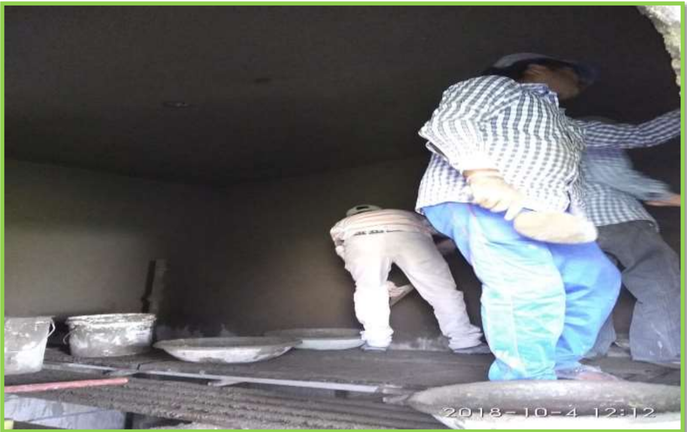
INTERNAL PLASTERING WORK
