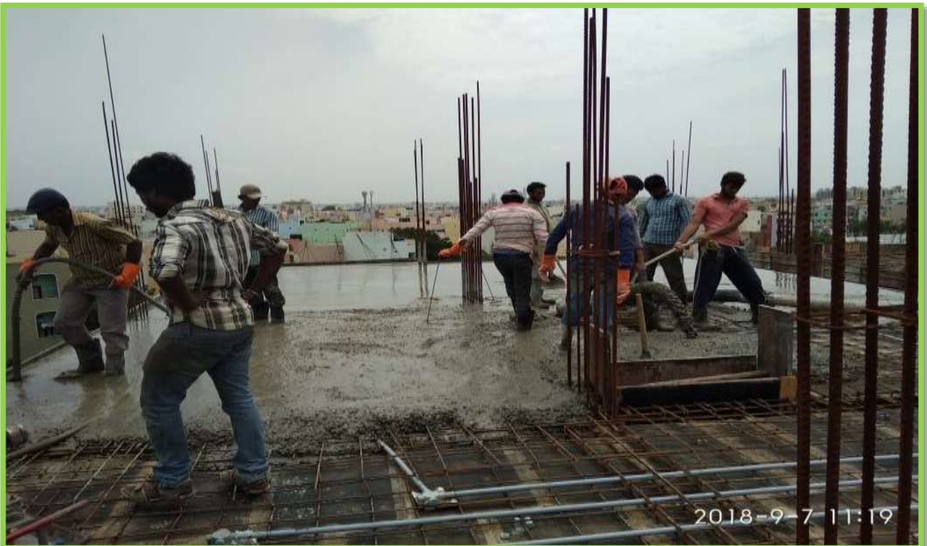
4 TH FLOOR SLAB CONCRETE WORK
