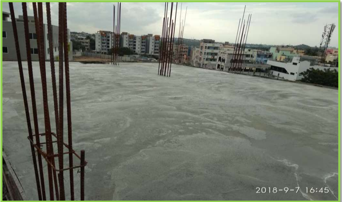
4 TH FLOOR SLAB CONCRETE WORK
