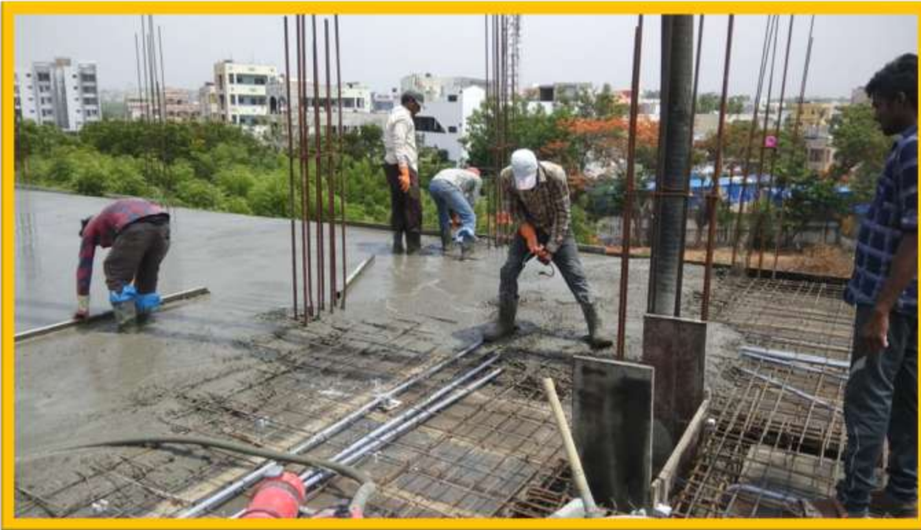
2 nd FLOOR SLAB CONCRETE WORK
