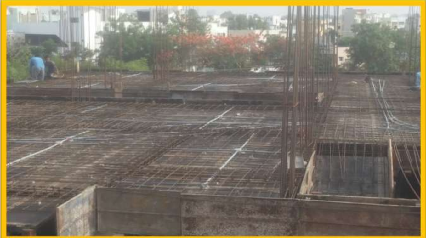
2 nd FLOOR SLAB SHUTTERING & BAR BENDING WORK
