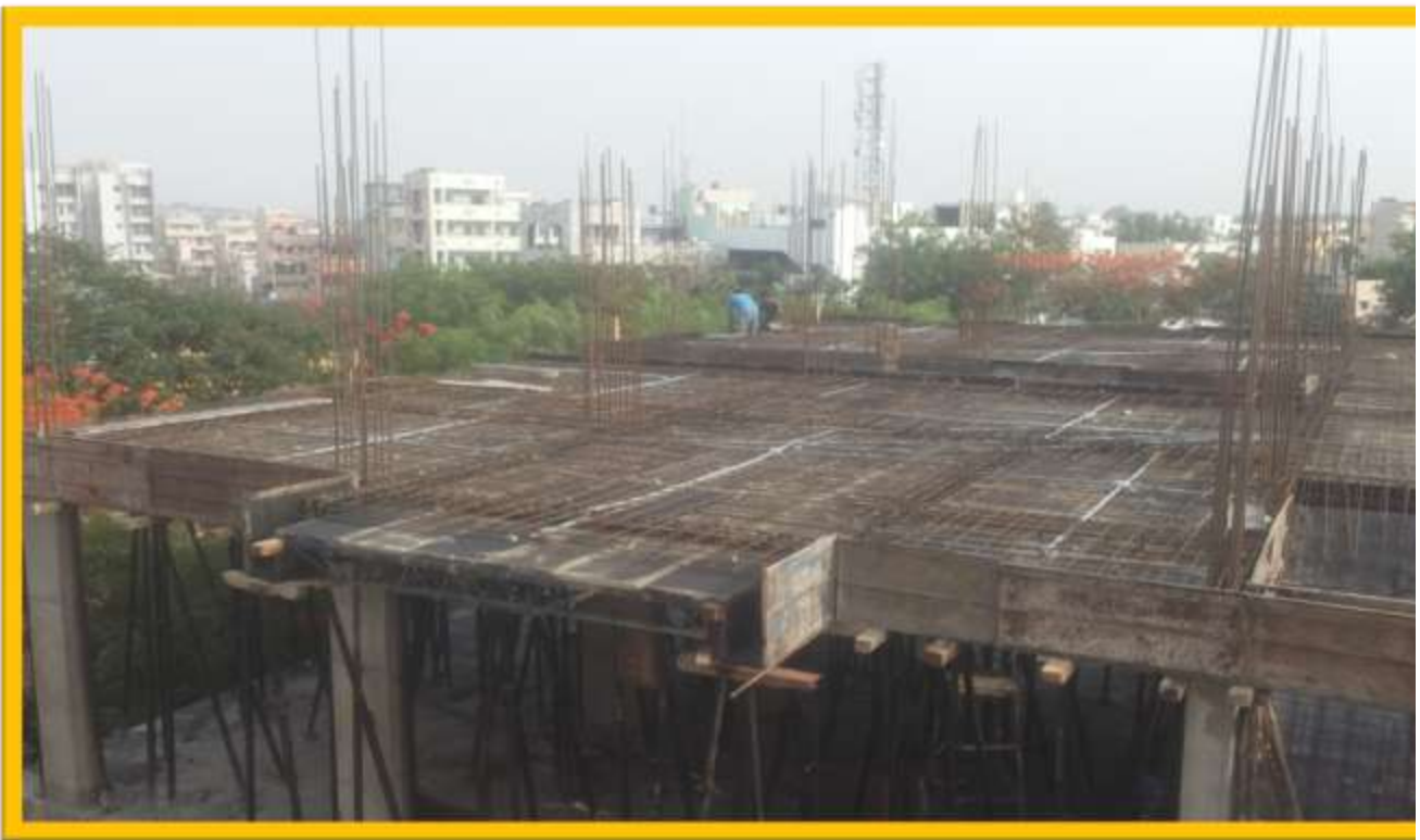
2 nd FLOOR SLAB SHUTTERING & BAR BENDING WORK
