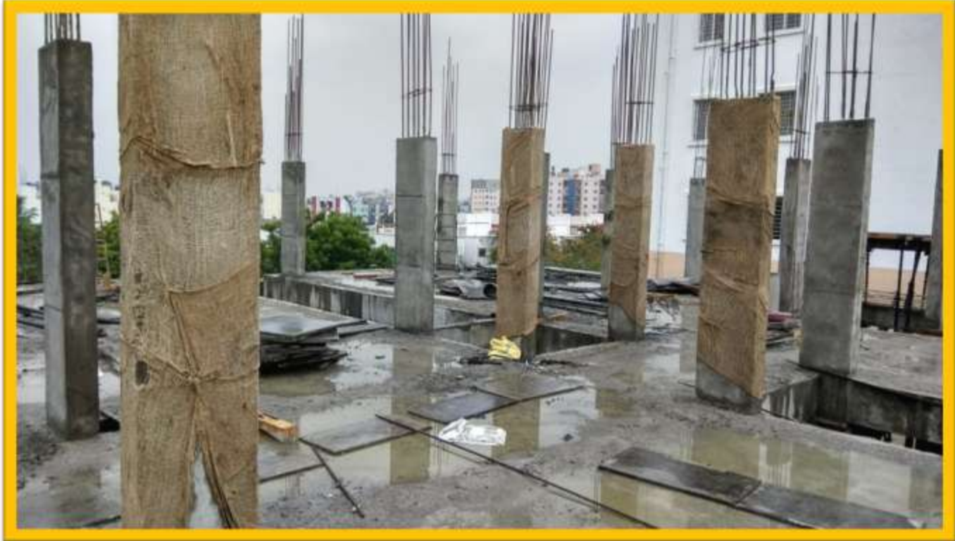
3 RD FLOOR COLUMNS CONCRETE WORK
