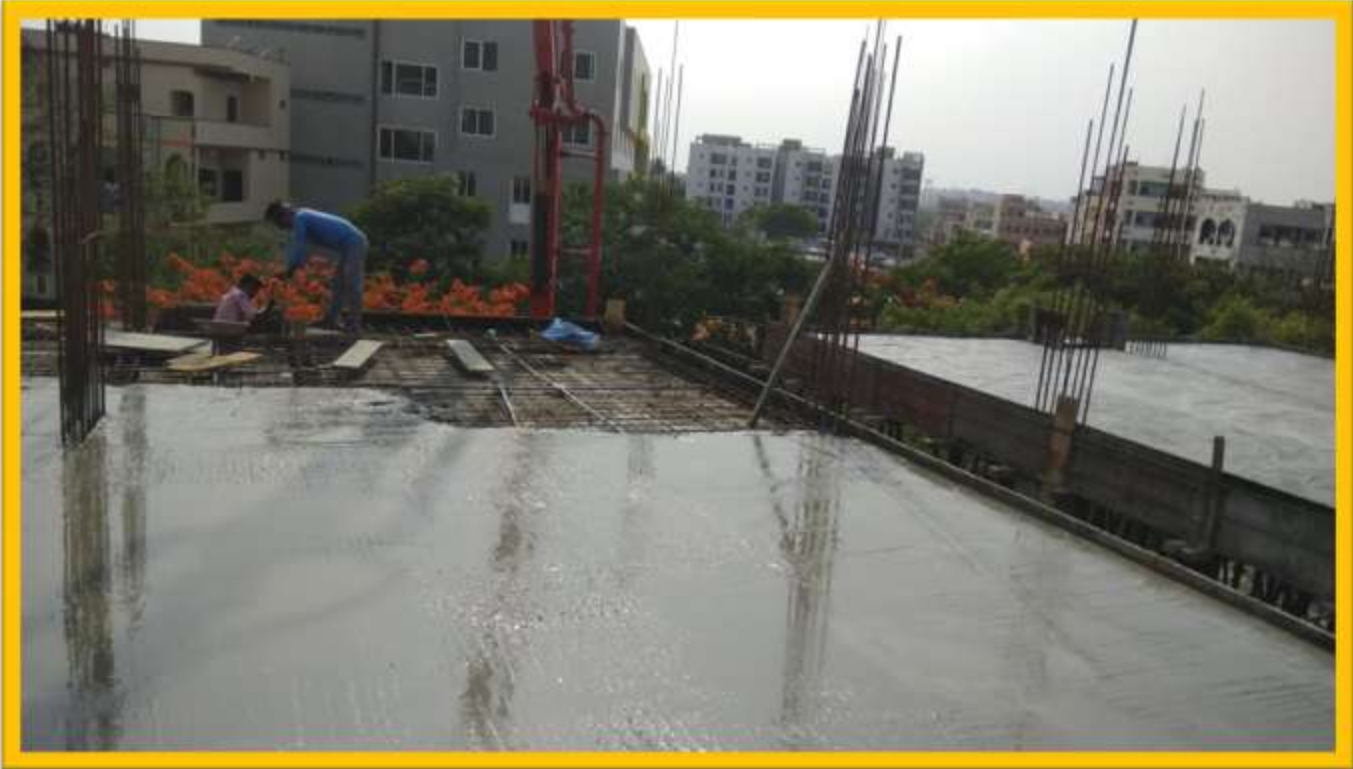
2 nd FLOOR SLAB CONCRETE WORK
