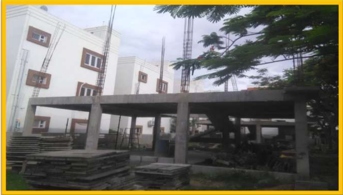
GROUND FLOOR SLAB AND 1 ST FLOOR COLUMNS STEEL OVERLAPPING
