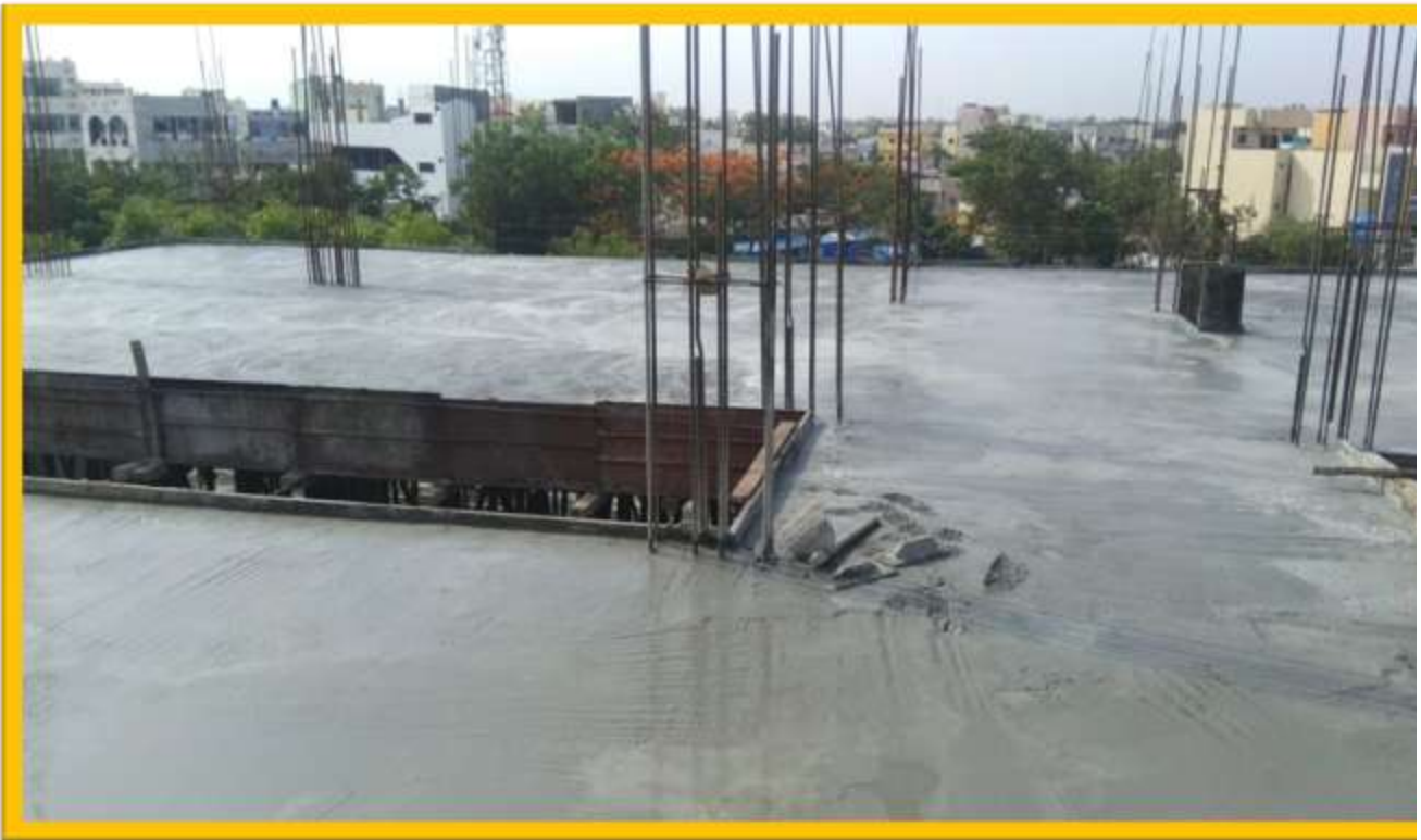
2 nd FLOOR SLAB CONCRETE WORK
