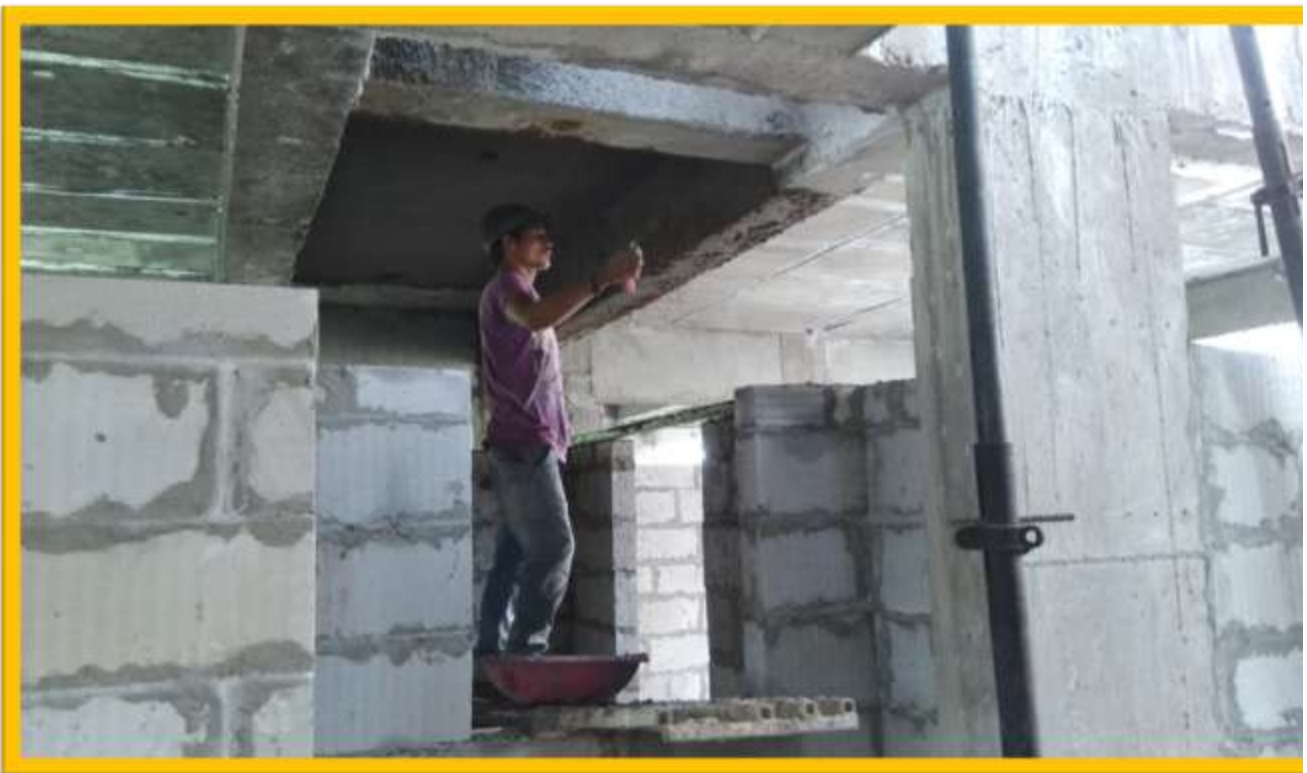
FIRST FLOOR BRICK WORK
