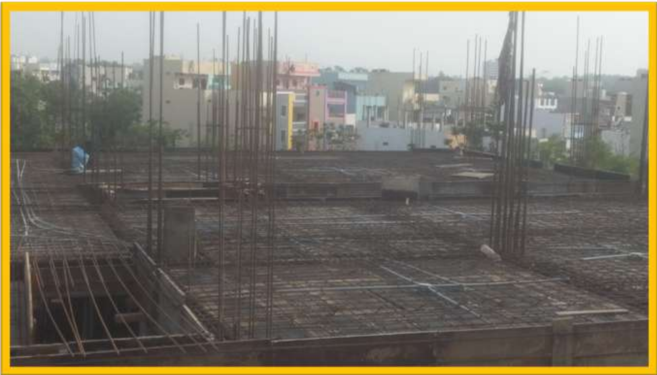
2 nd FLOOR SLAB SHUTTERING & BAR BENDING WORK
