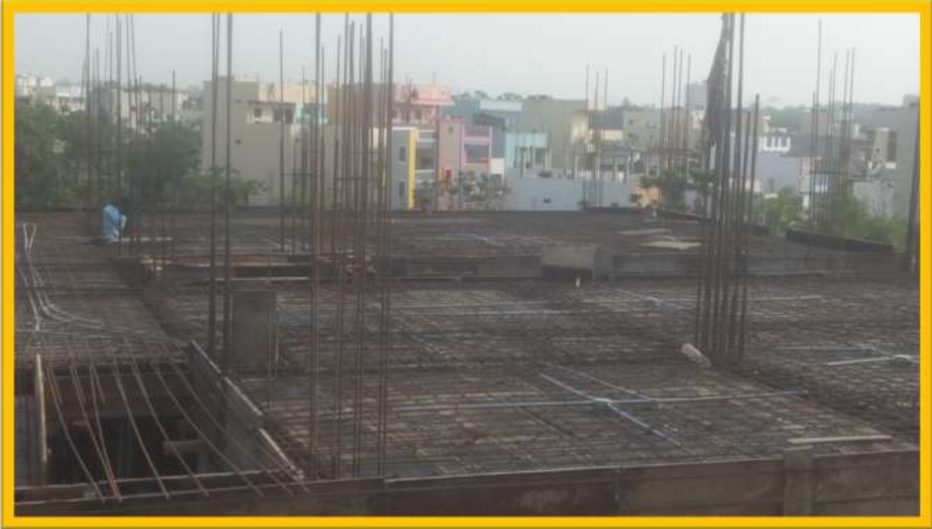
2 nd FLOOR SLAB SHUTTERING & BAR BENDING WORK
