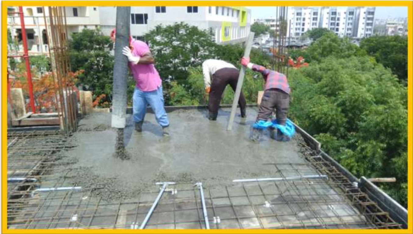
2 nd FLOOR SLAB CONCRETE WORK
