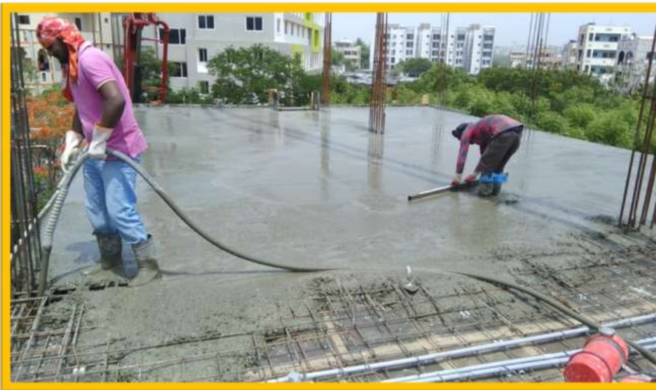
2 nd FLOOR SLAB CONCRETE WORK
