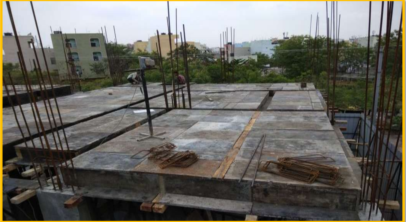
2 nd SLAB SHUTTERING WORK
