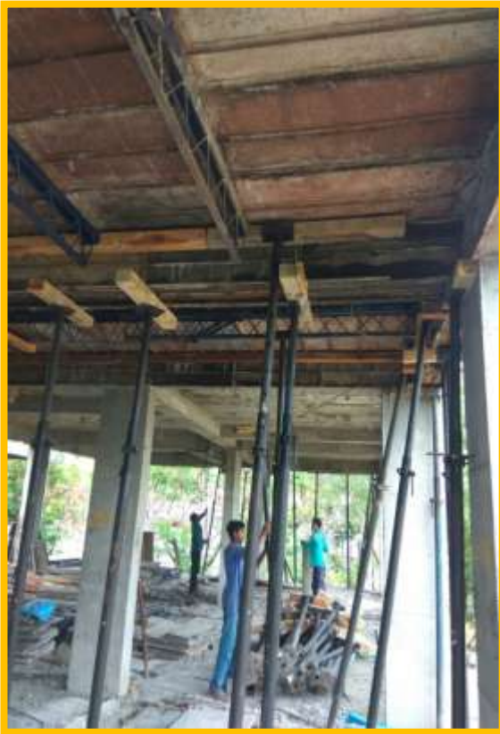
2 ND SLAB DE- SHUTTERING WORK
