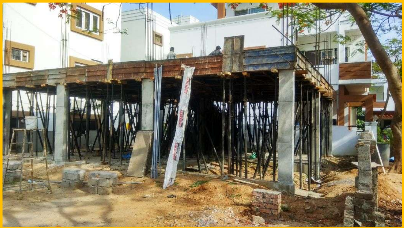
SLAB SHUTTERING AND BAR BENDING WORK
