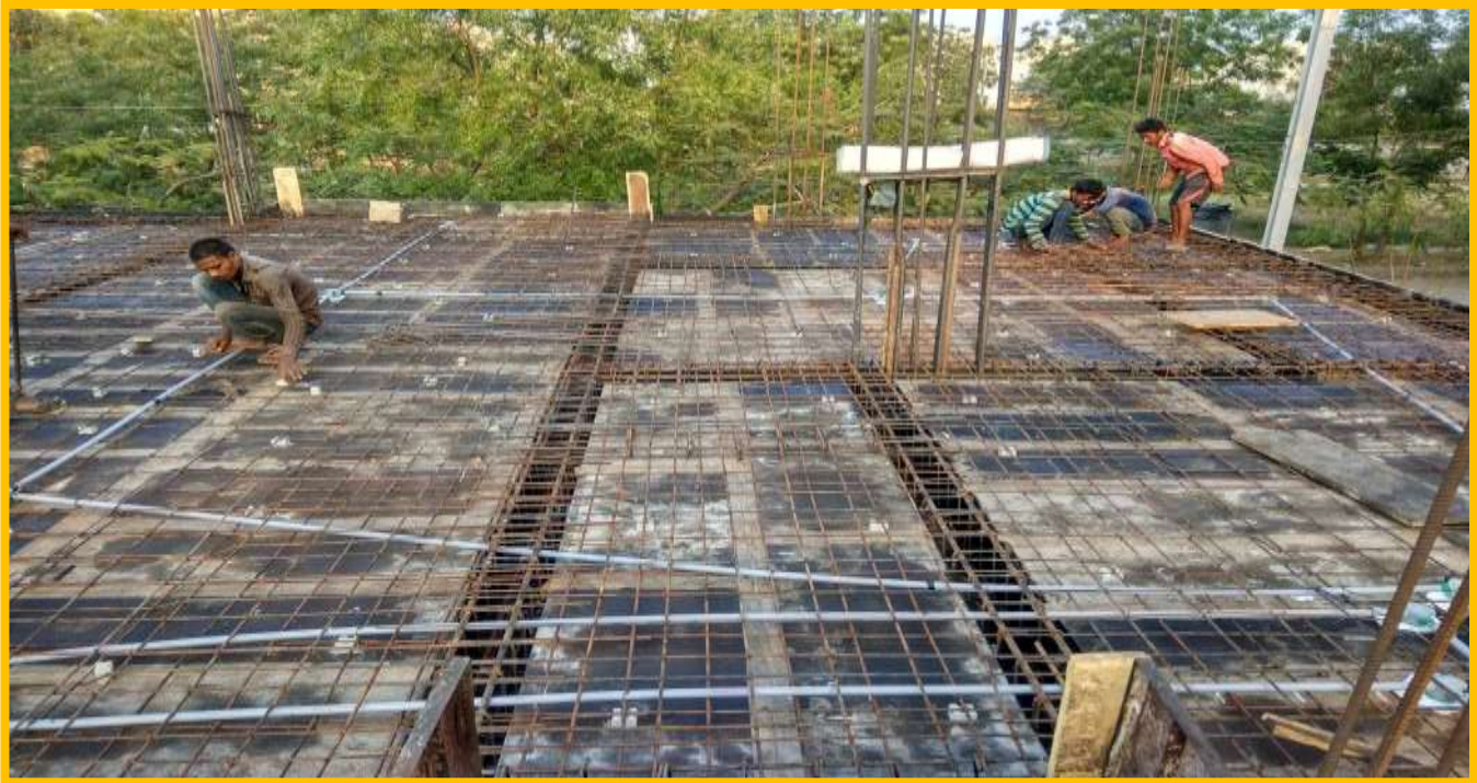
2 nd SLAB BAR BENDING WORK
