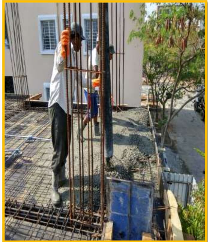
2 nd SLAB CONCRETE WORK WITH BOOMER MACHINE
