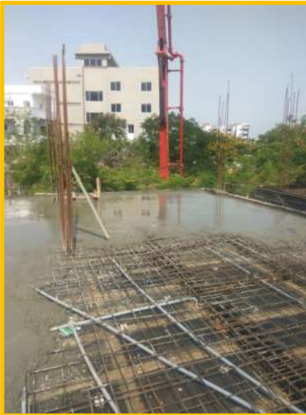
2 nd SLAB CONCRETE WORK WITH BOOMER MACHINE
