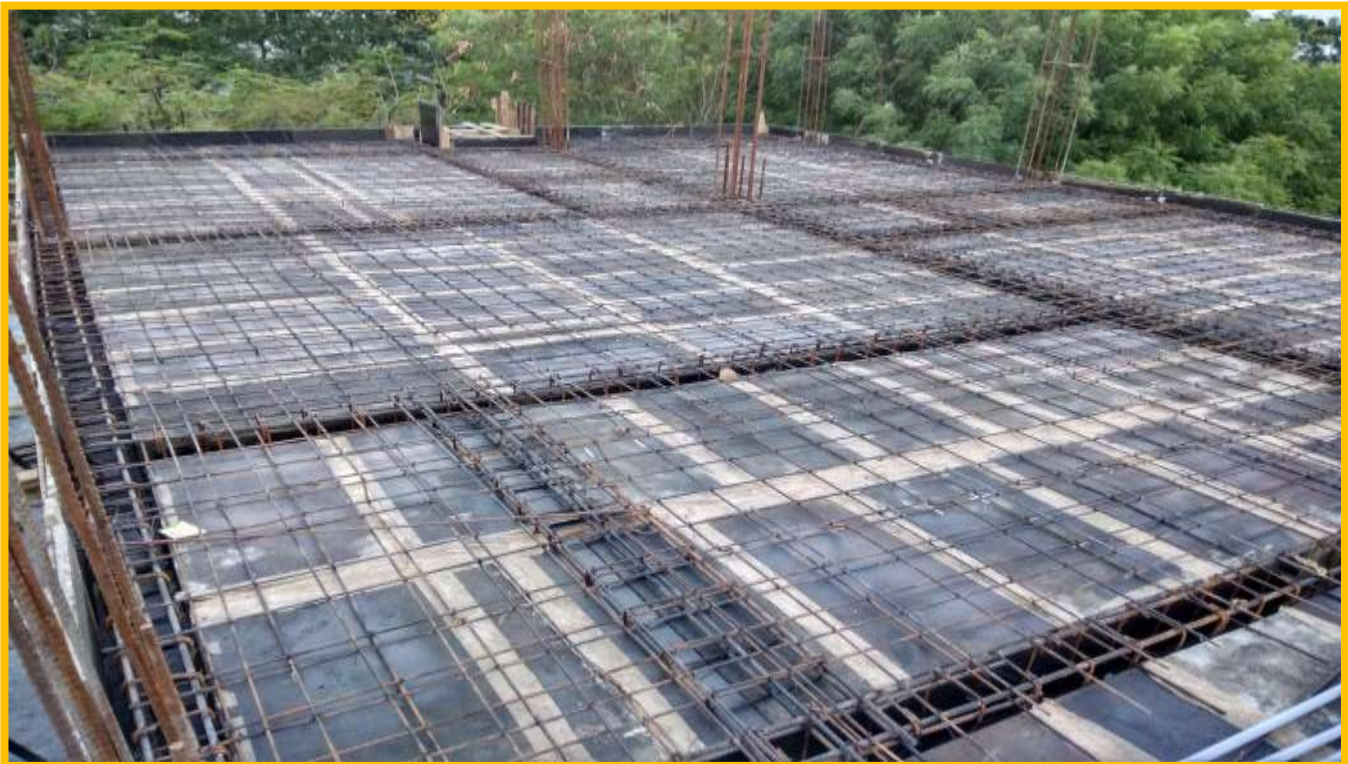
2 nd SLAB BAR BENDING WORK
