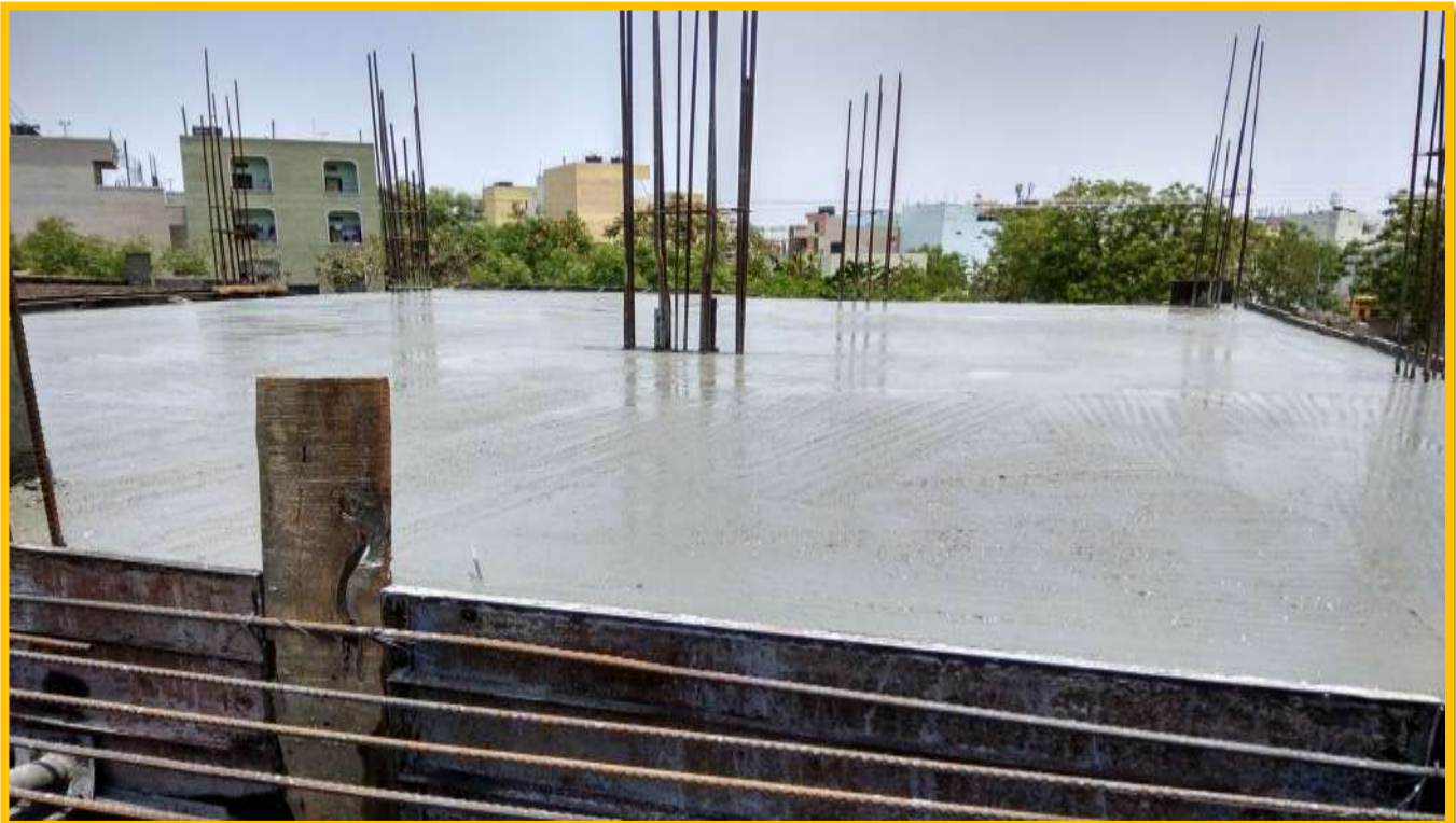
2 nd SLAB CONCRETE WORK
