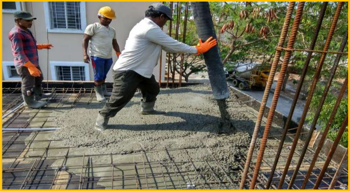
2 nd SLAB CONCRETE WORK
