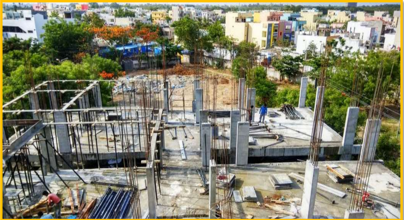
3 RD SLAB SHUTTERING WORK IN PROGRESS
