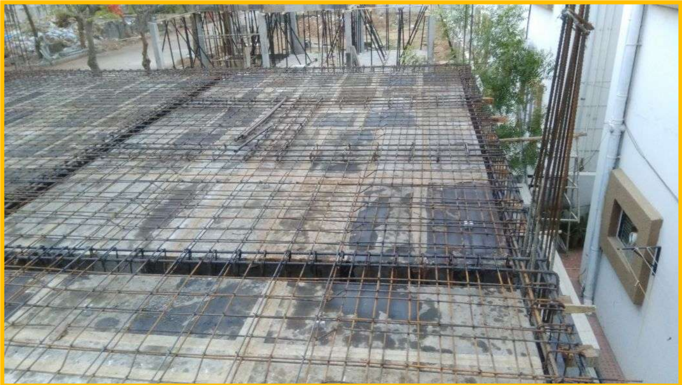
SLAB SHUTTERING AND BAR BENDING WORK
