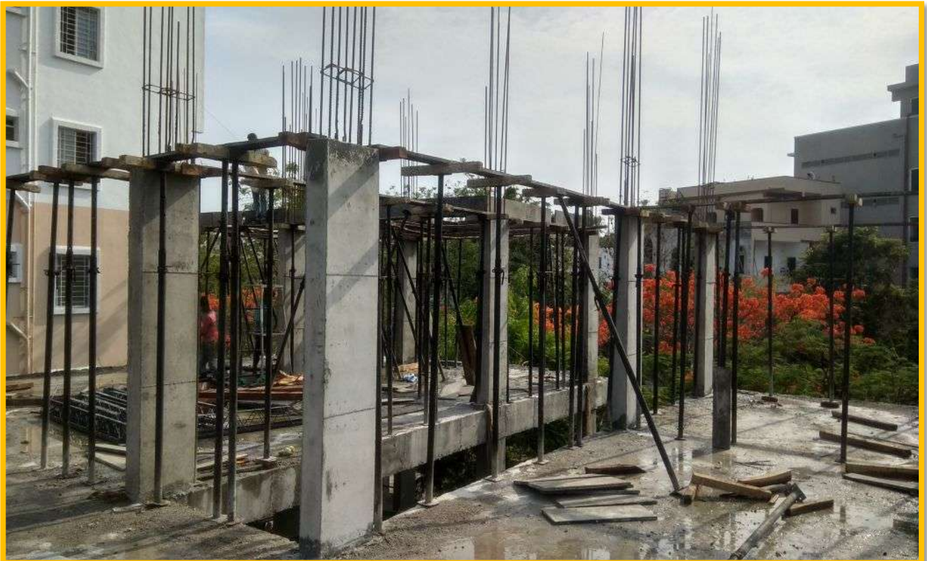
3 RD SLAB SHUTTERING WORK IN PROGRESS
