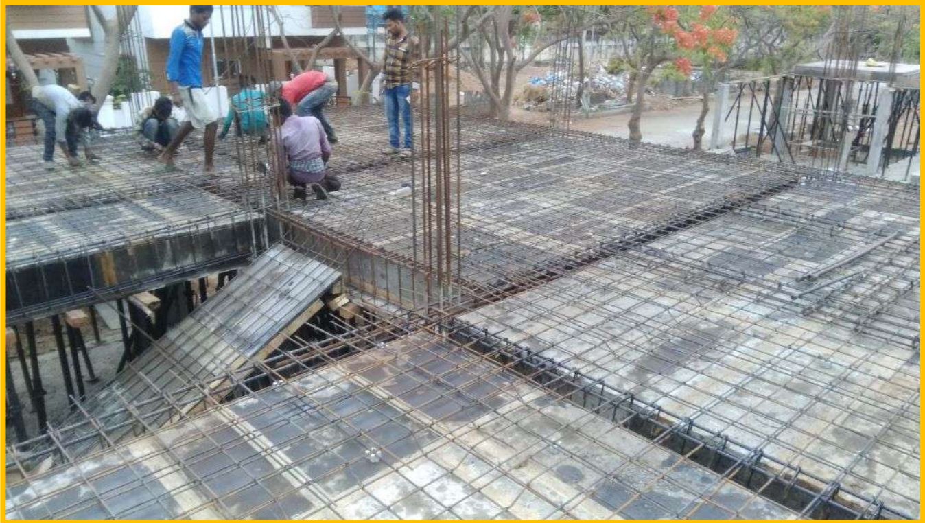
SLAB SHUTTERING AND BAR BENDING WORK
