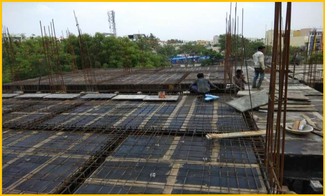
2 nd SLAB BAR BENDING WORK
