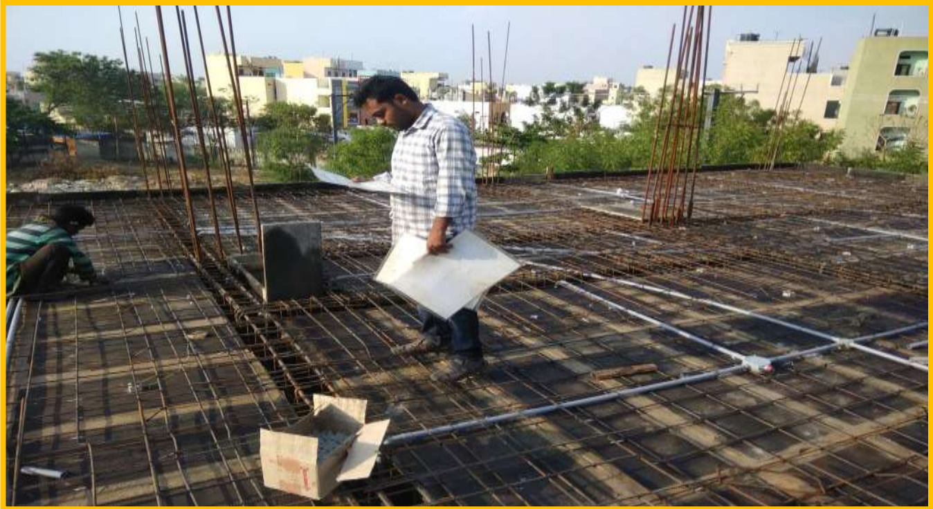
2 nd SLAB BAR BENDING CHECKING WORK STRUCTURAL CONSUTANT
