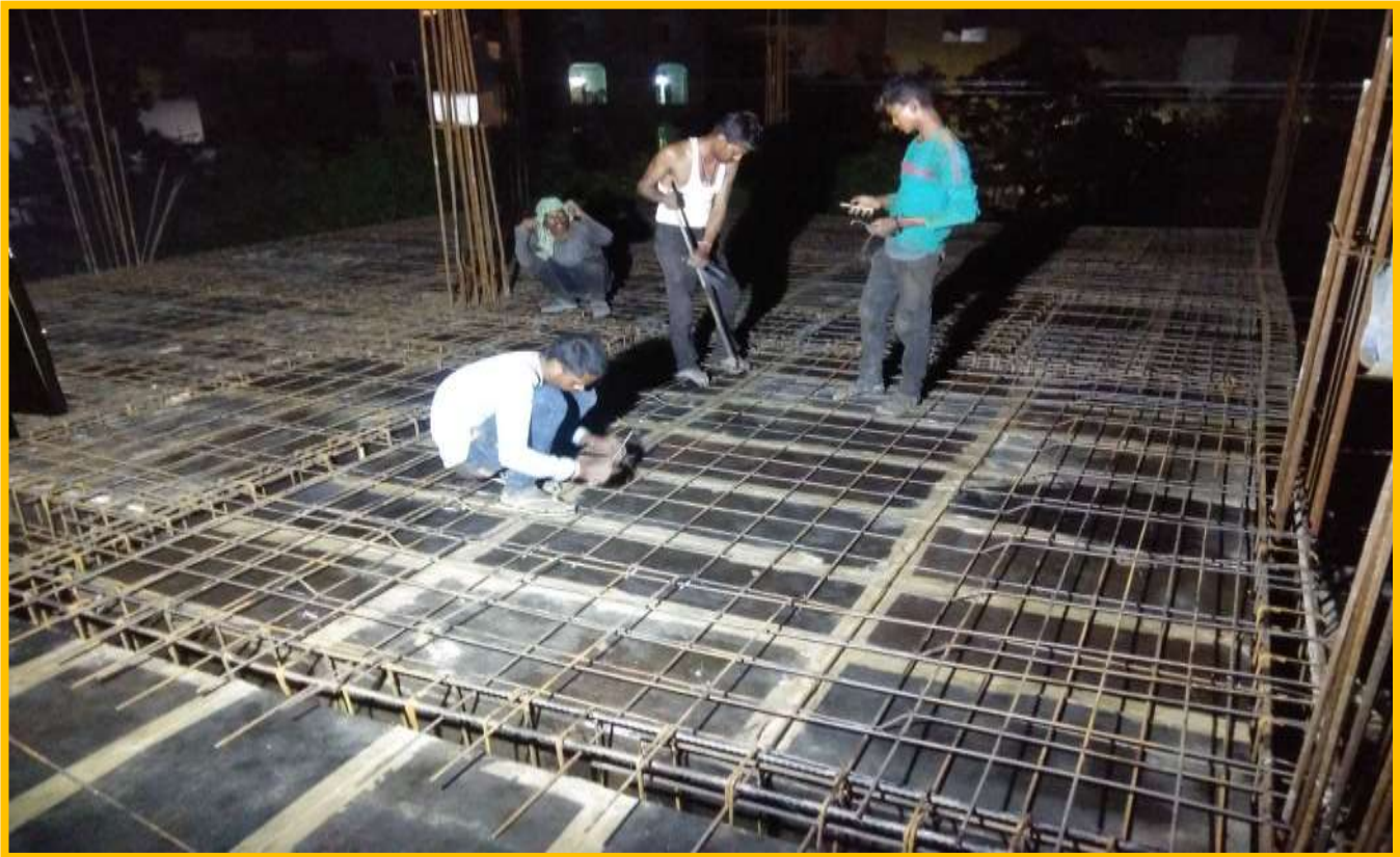
2 nd SLAB BAR BENDING WORK
