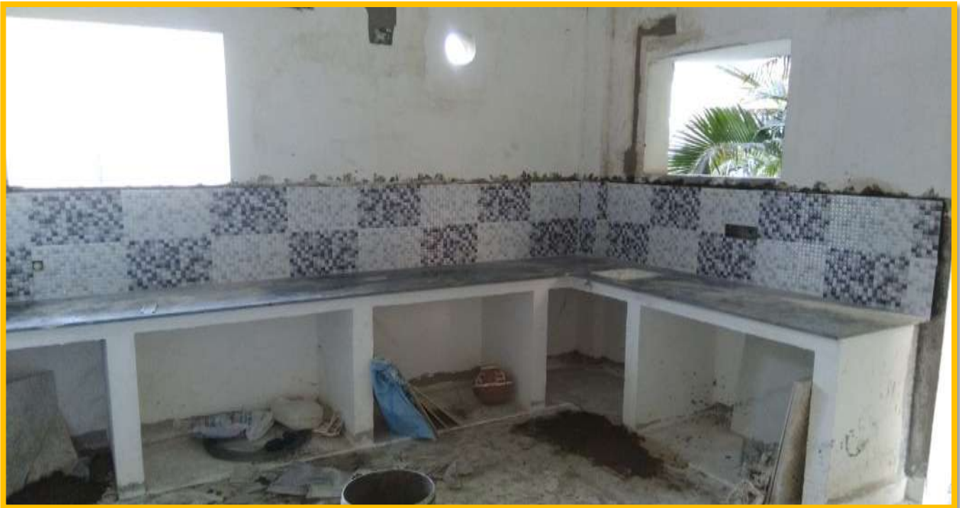
KITCHEN/PARKING AND TERRACE TILES LAYING WORK
