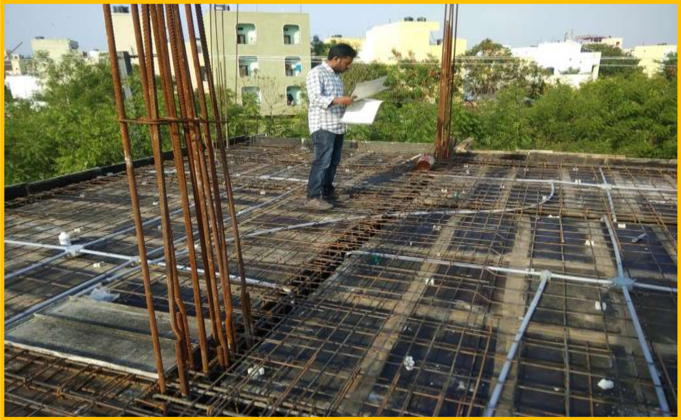
2 nd SLAB BAR BENDING CHECKING WORK STRUCTURAL CONSUTANT
