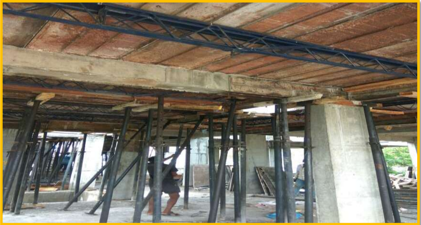
2 ND SLAB DE- SHUTTERING WORK
