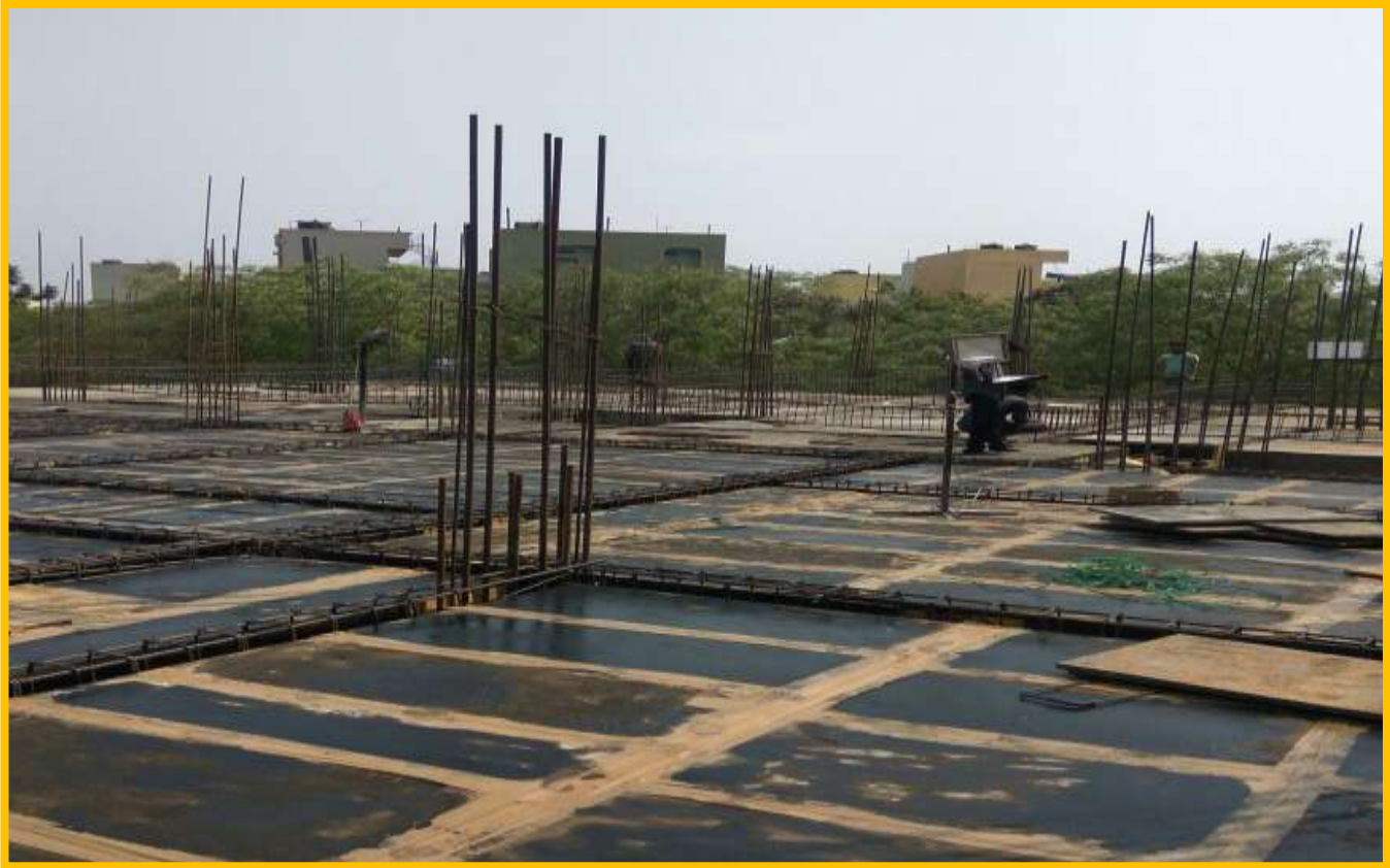
2 nd SLAB SHUTTERING WORK
