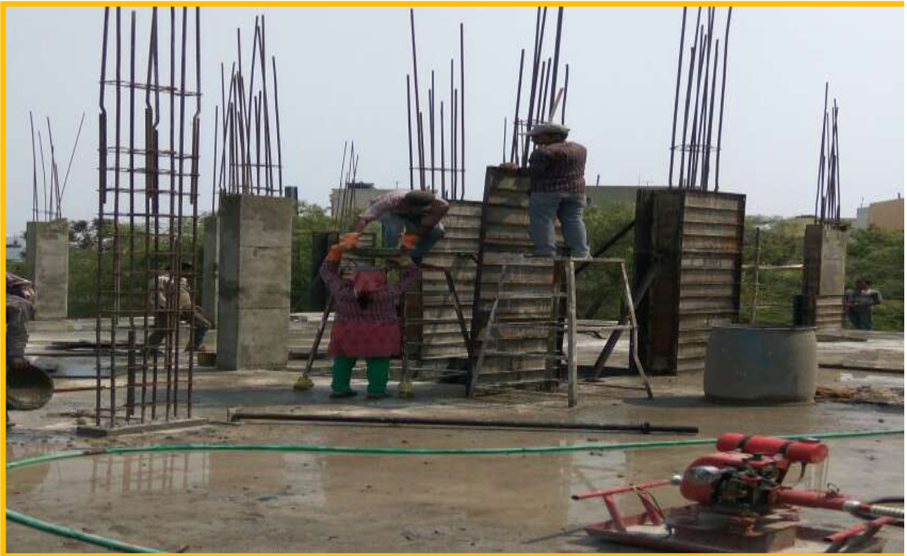
3 RD SLAB COUMNS CONCRETE WORK
