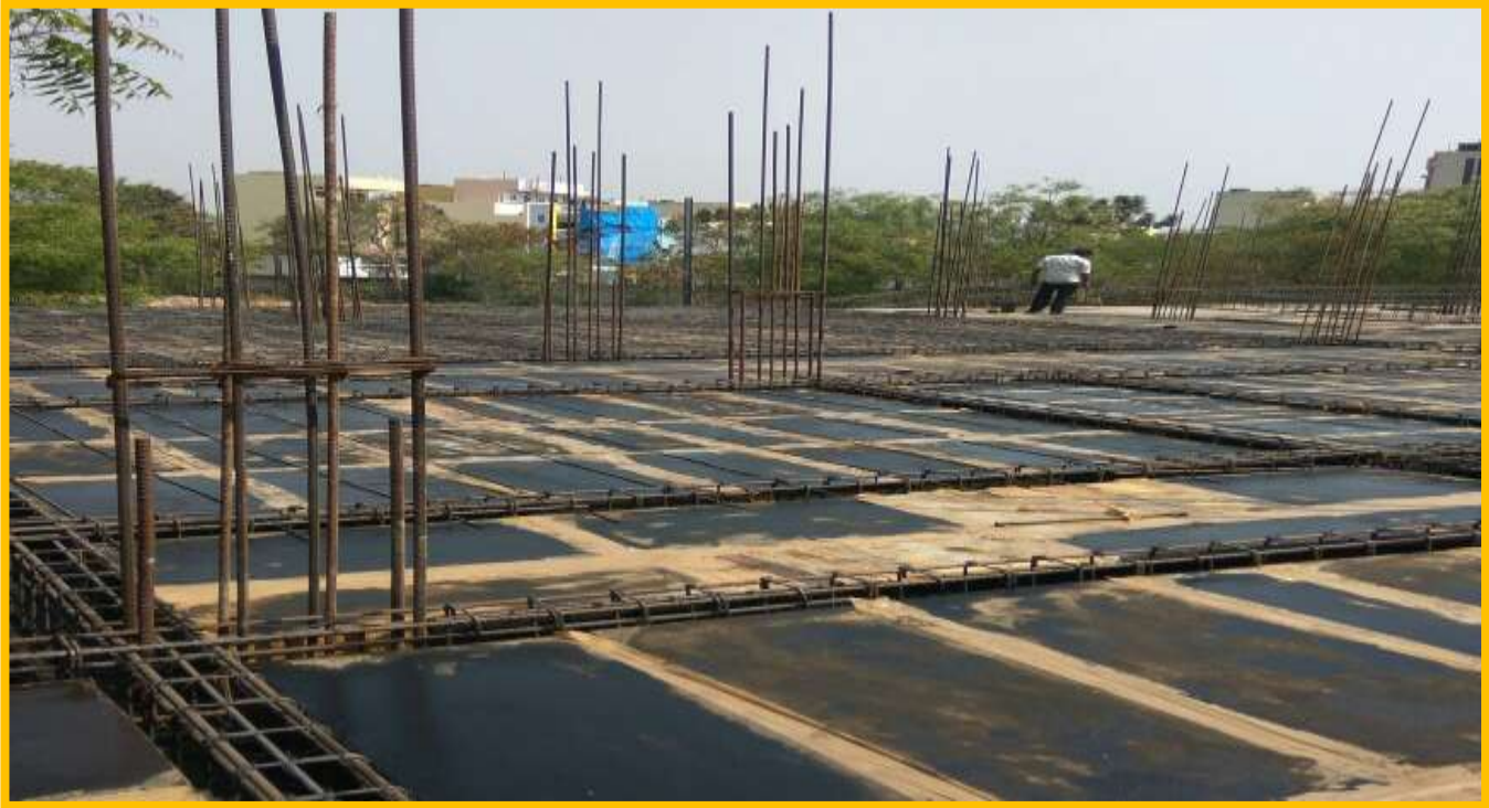
2 nd SLAB SHUTTERING WORK
