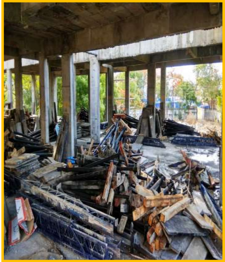
2 ND SLAB DE- SHUTTERING WORK
