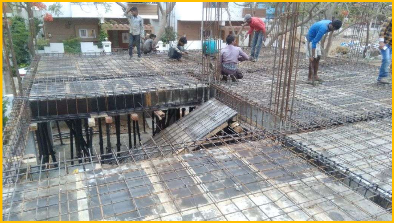
SLAB SHUTTERING AND BAR BENDING WORK
