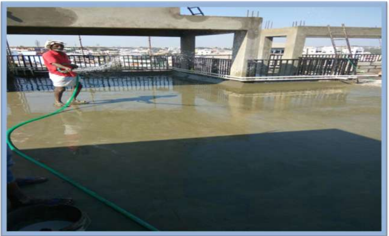
WATER PROOFING AT TERRACE AREA
