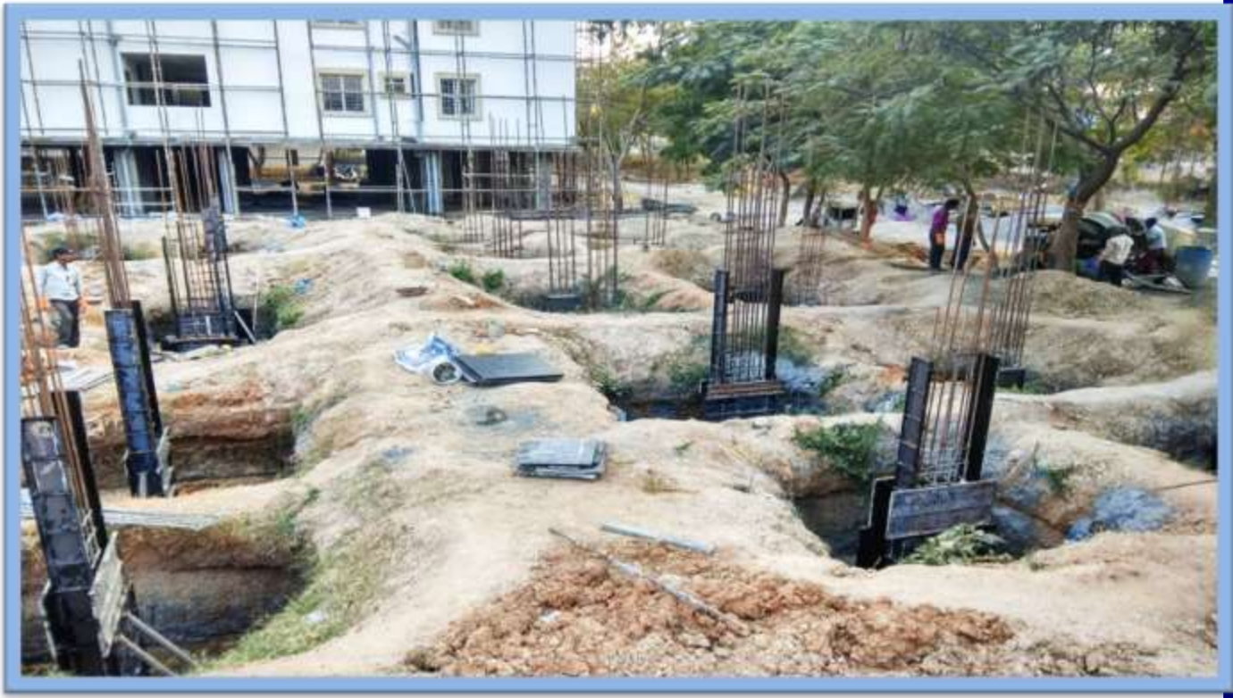
PEDESTAL CONCRETE WORK COMPLETED
