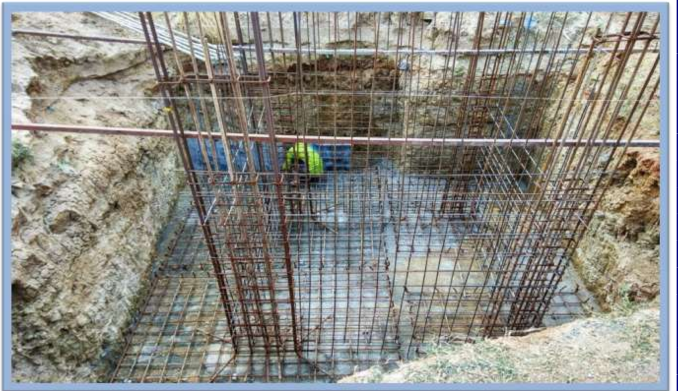
LIFT PIT FOOTING AND COLUMNS MATS
