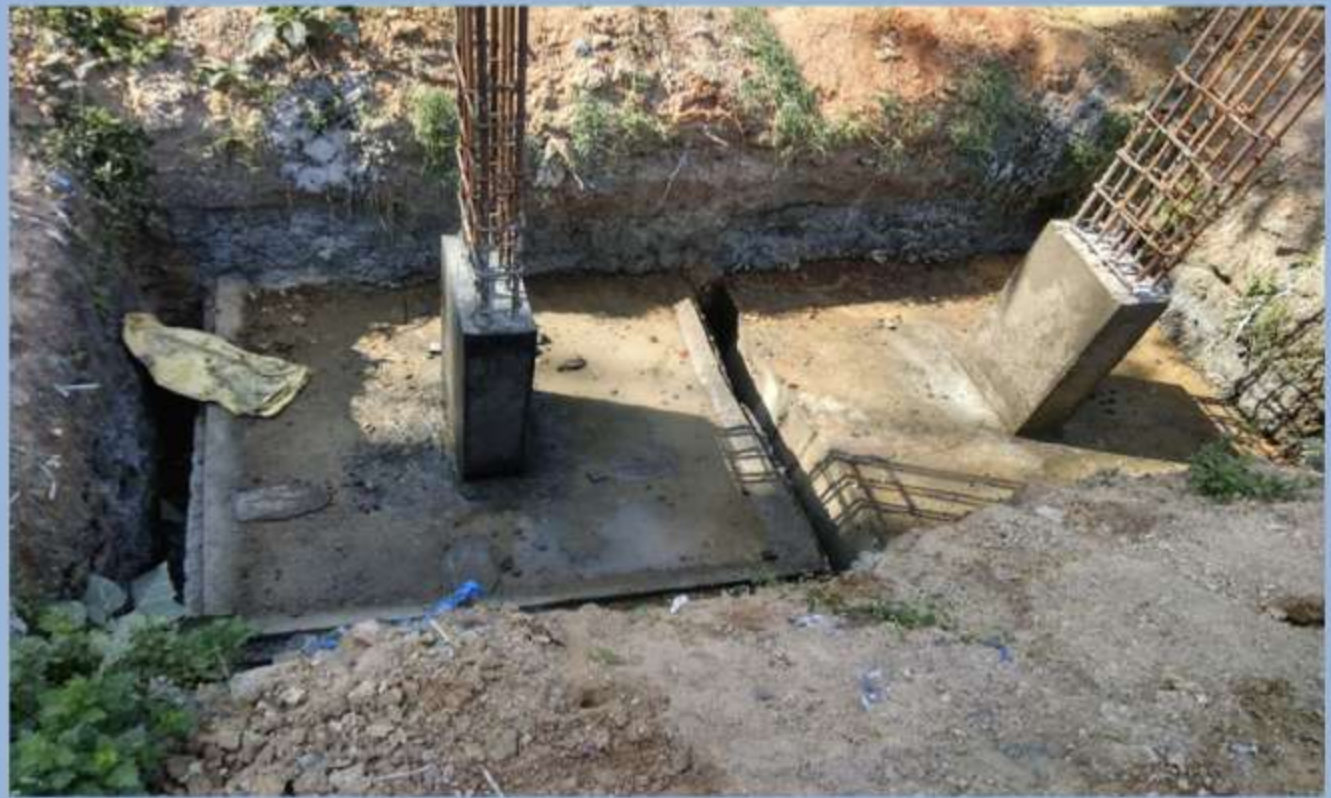
PEDESTAL CONCRETE WORK COMPLETED
