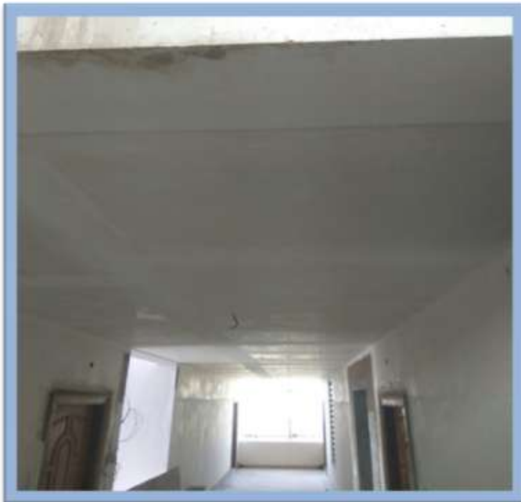
FALSE CEILING AT CORRIDOR AREA
