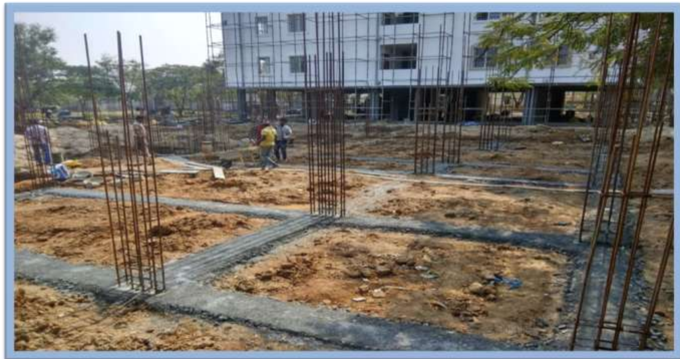
P.C.C. WORK FOR PLINTH BEAM PURPOSE
