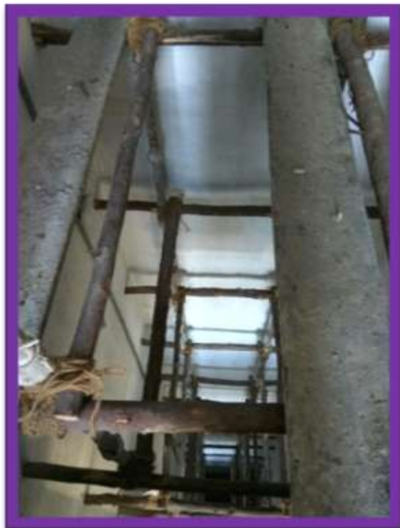
SCAFFOLDING AND HOOK WORK COMPLETED FOR LIFT WORK PURPOSE.
