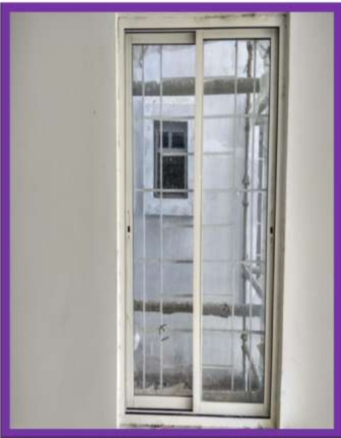
ALUMINUM FRAME & SHUTTER FIXING WORK
