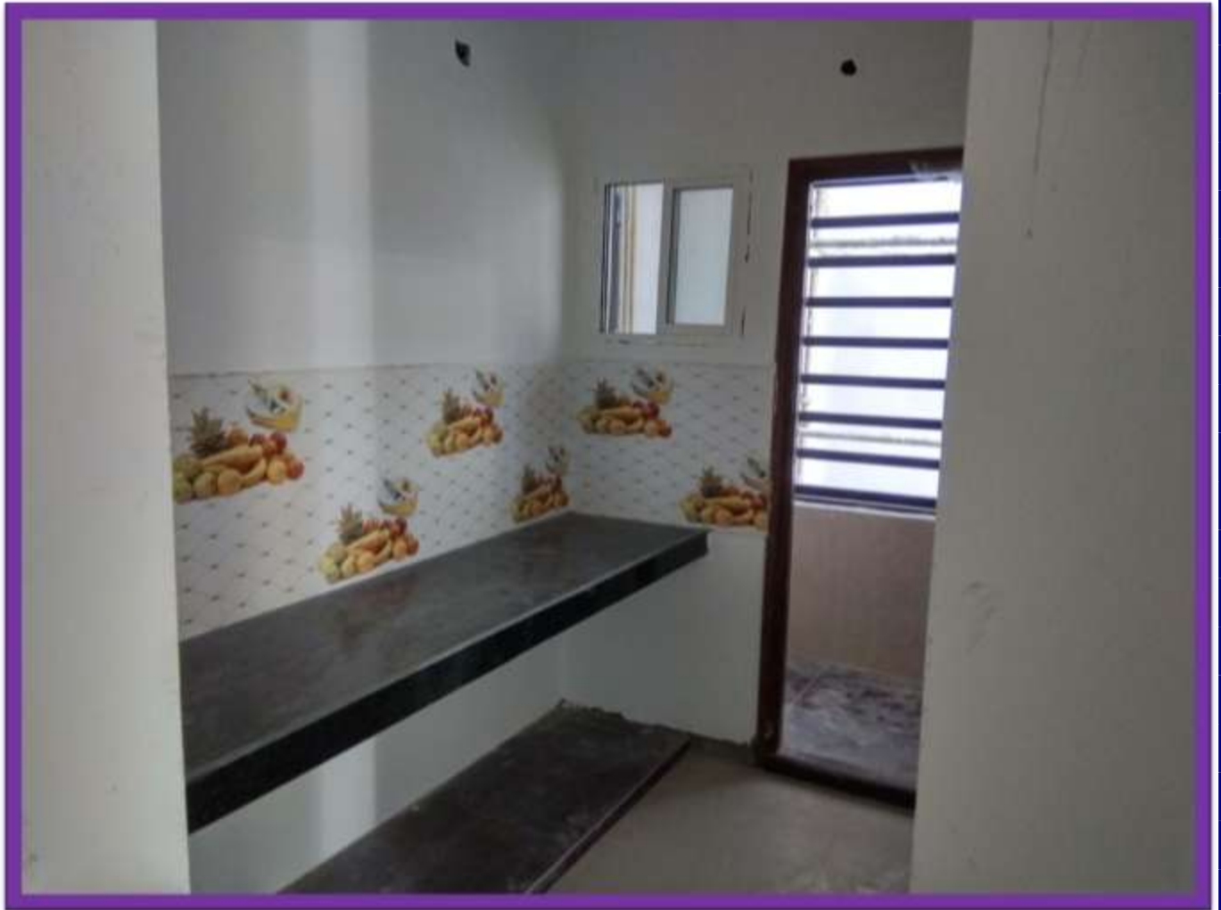
KITCHEN WALL DADO AND GRANITE PLATFORM WORK
