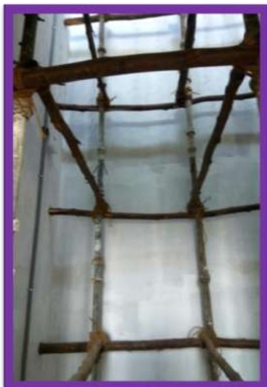
SCAFFOLDING AND HOOK WORK COMPLETED FOR LIFT WORK PURPOSE.
