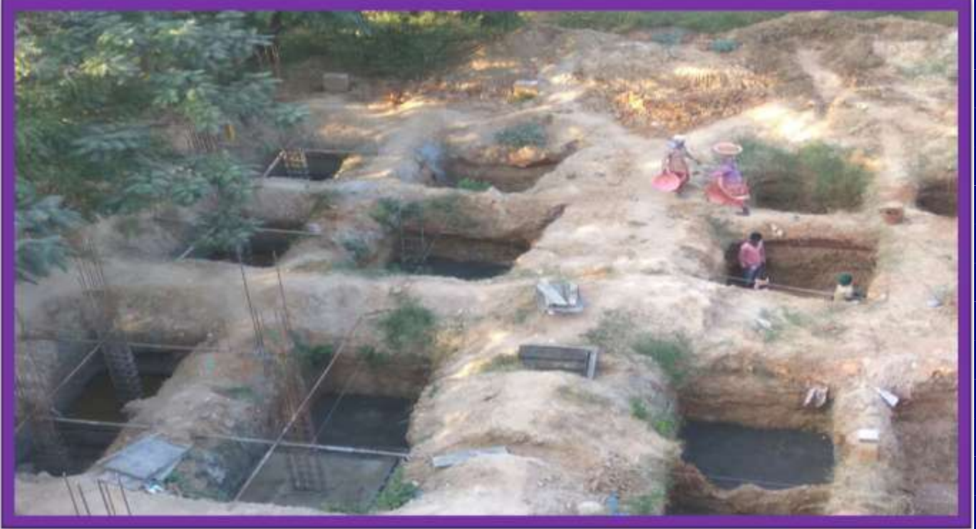
FOOTING AND P.C.C CONCRETE WORK
