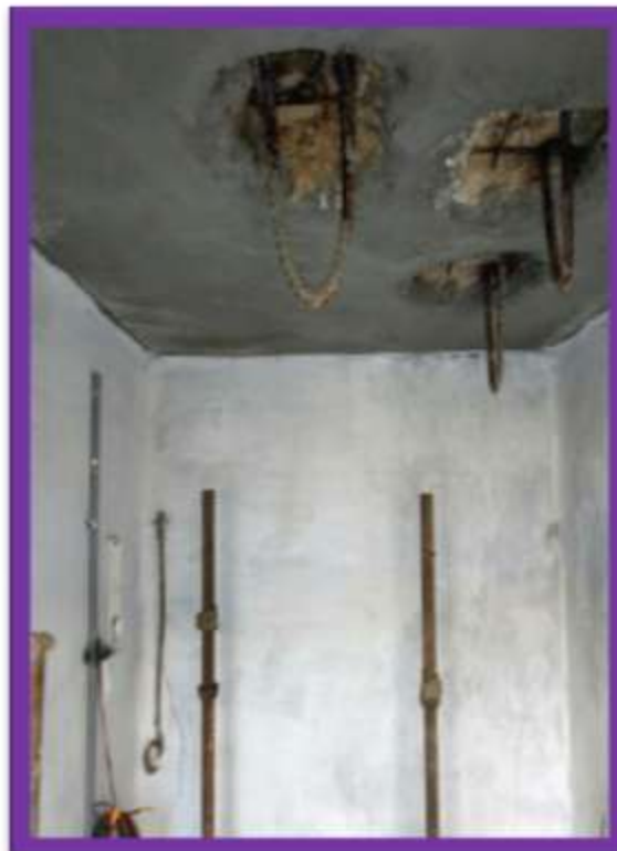
SCAFFOLDING AND HOOK WORK COMPLETED FOR LIFT WORK PURPOSE.
