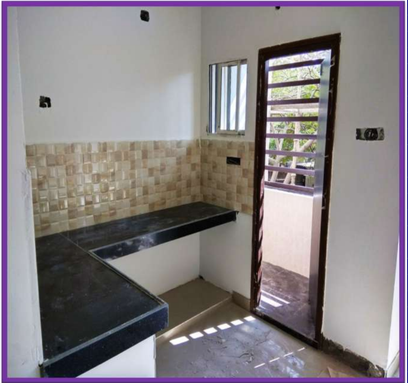
KITCHEN WALL DADO AND GRANITE PLATFORM WORK
