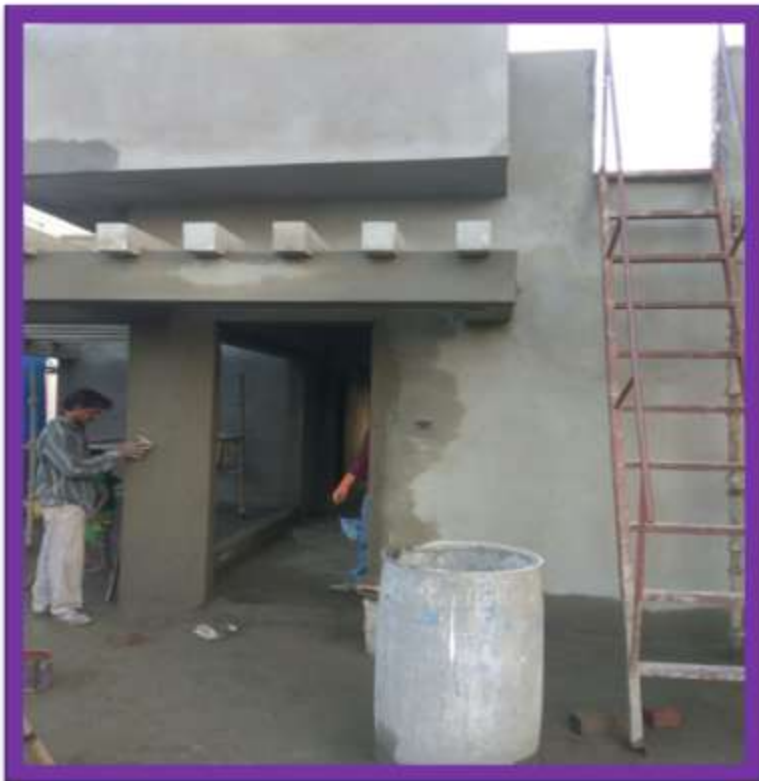
Terrace Pergola Elevation plastering work
