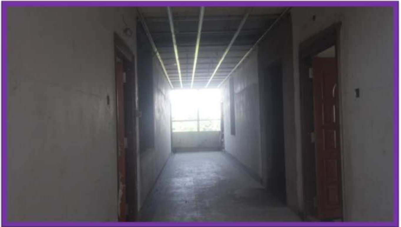
AluminumChannel for False Ceiling fixing work completed.
