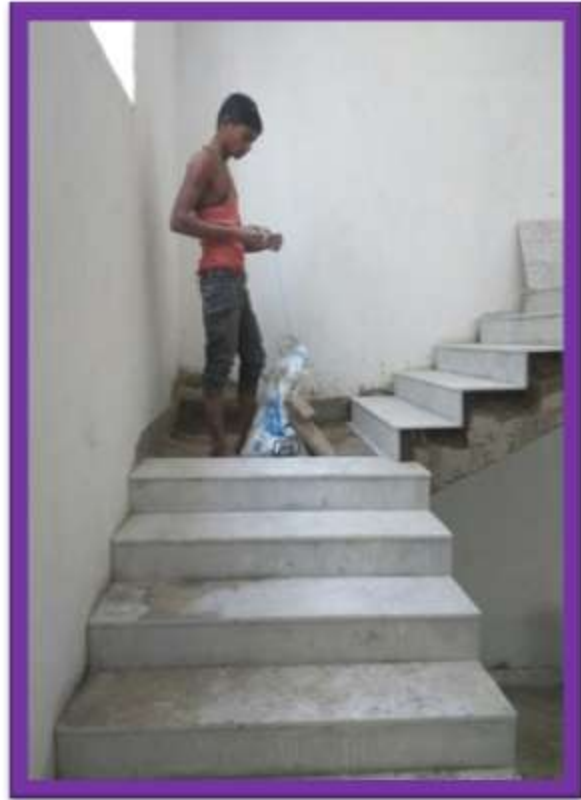
Marble Laying work in progress.
