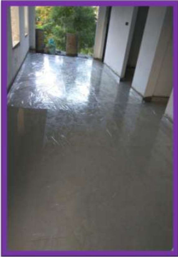
5 th Floor All Flats Vitrified Tiles laying work completed.
